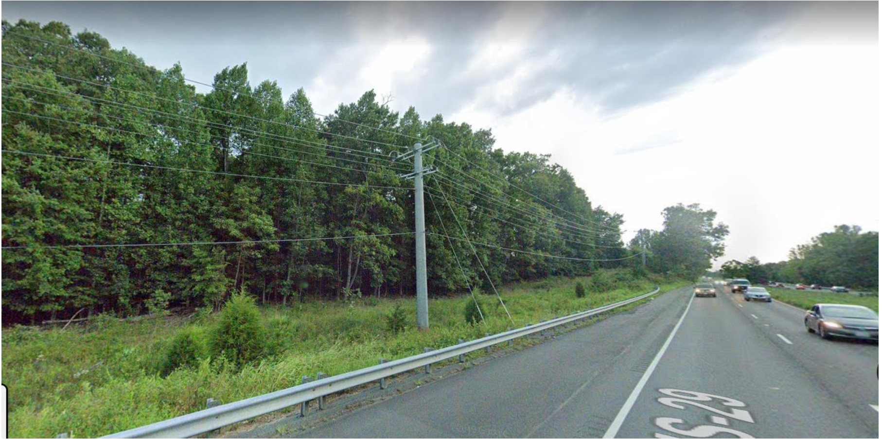
Figure 4b: Google street view looking north showing a representative frontage condition along the corridor with wooded area, cleared frontage, and an open view of the power lines.
