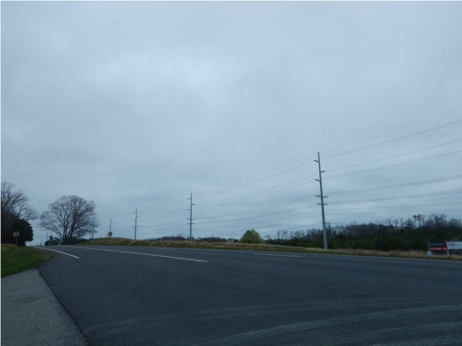
Figure 1: View of completed power line upgrade in Greene County.
