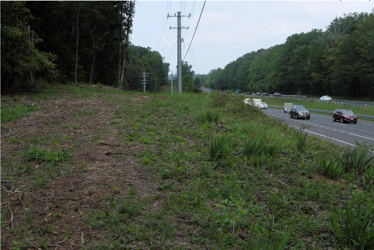
View north from Frays Mill Road
