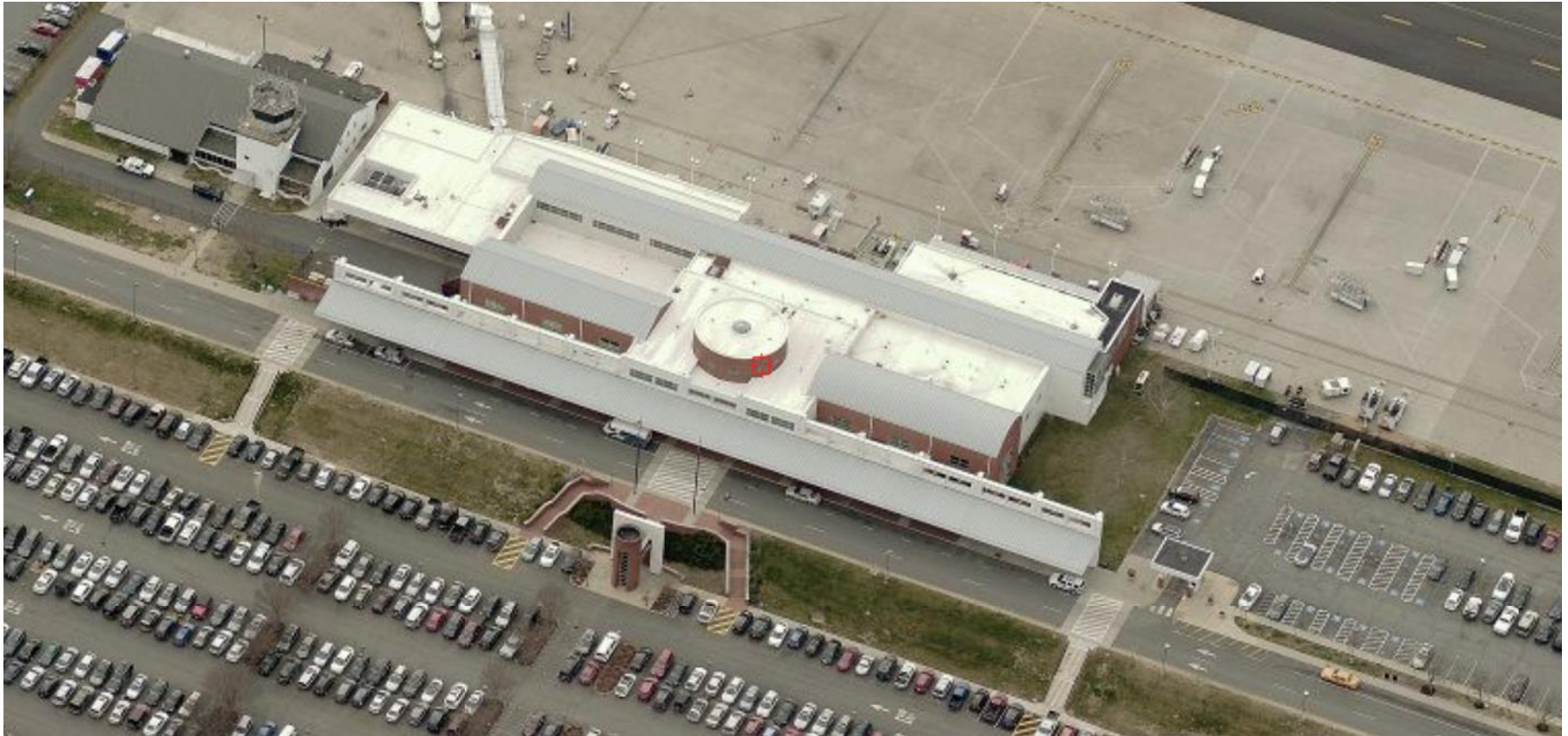
Figure 1: Aerial view of the main terminal building with the existing central elevator and stairs, and stairs at the north and south ends of the canopy.
