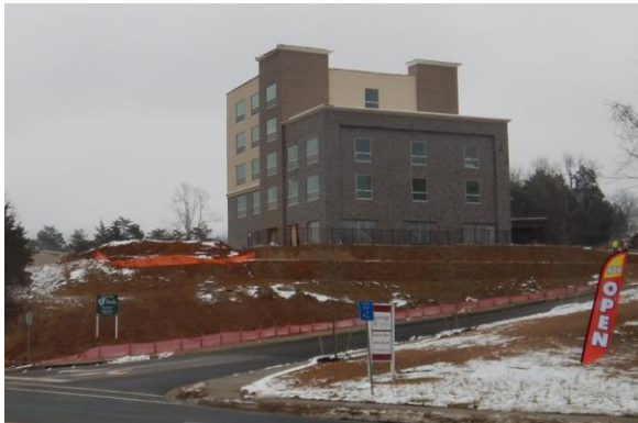
Figure 1c: View of west elevation under construction (February 2021).
