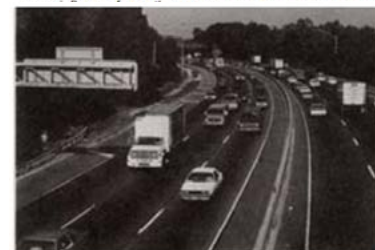
Level of Service C: Restricted flow that remains stable but with significant interactions with others in the traffic stream. The general level of comfort and convenience declines noticeably at this level.
