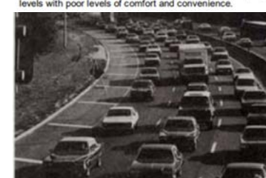
Level of Service F: Forced traffic flow in which the amount of traffic approaching a point exceeds the amount that can be served. LOS F is characterized by stop-and-go waves, poor travel times, low comfort and convenience, and
