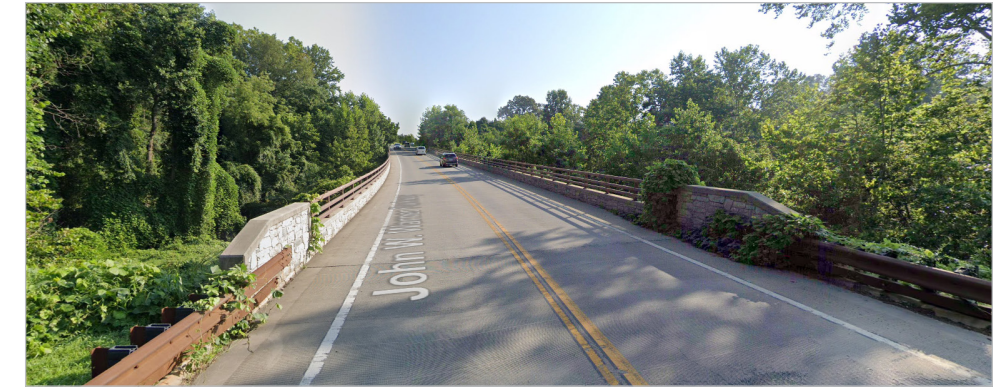
Stone veneer on the corridor's bridges supports the natural aesthetic of the Parkway.
