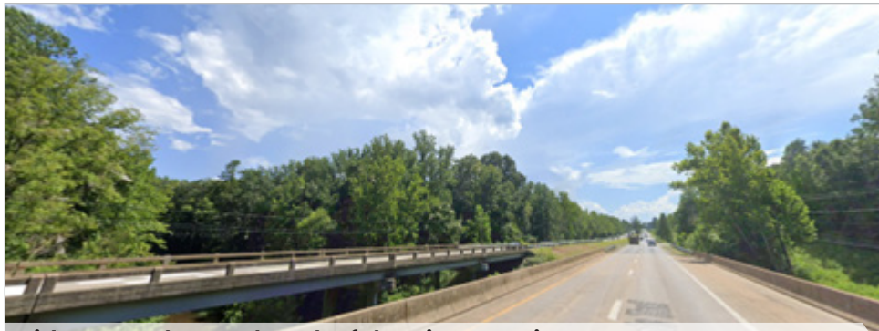
Bridge over the North Fork of the Rivanna River
