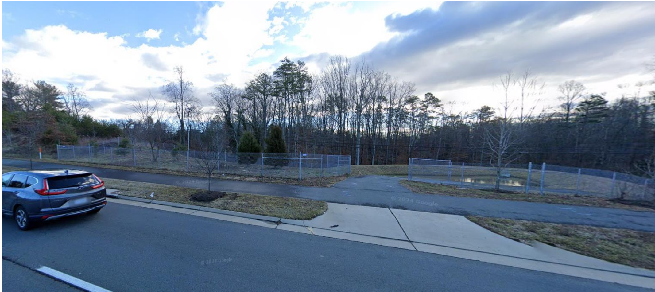
Figure 3: View looking east from Rt. 29 near the VDOT stormwater facility.
