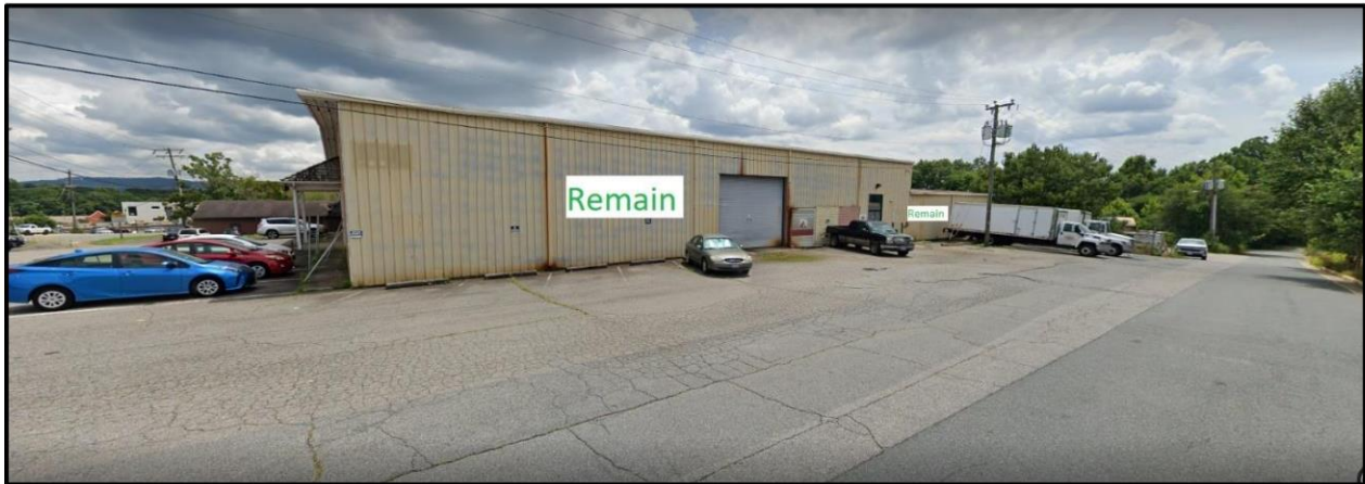
Side View from Shared Street with Northside Library
