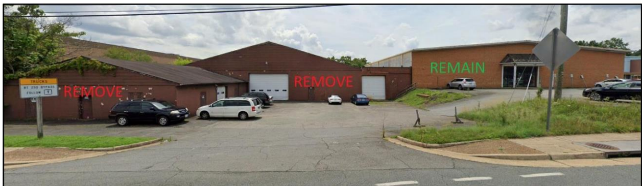
Front View from Rio Rd
