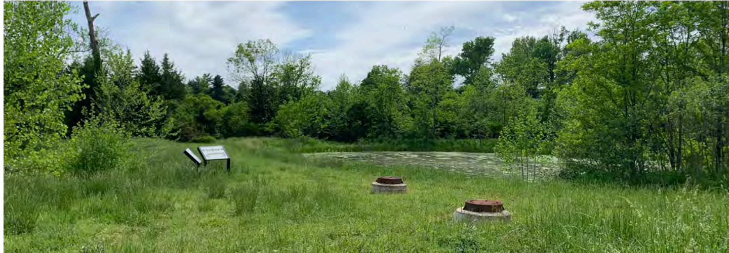
The existing County-owned stormwater management facility recommended for enhancement to provide a trail access point is pictured above.
