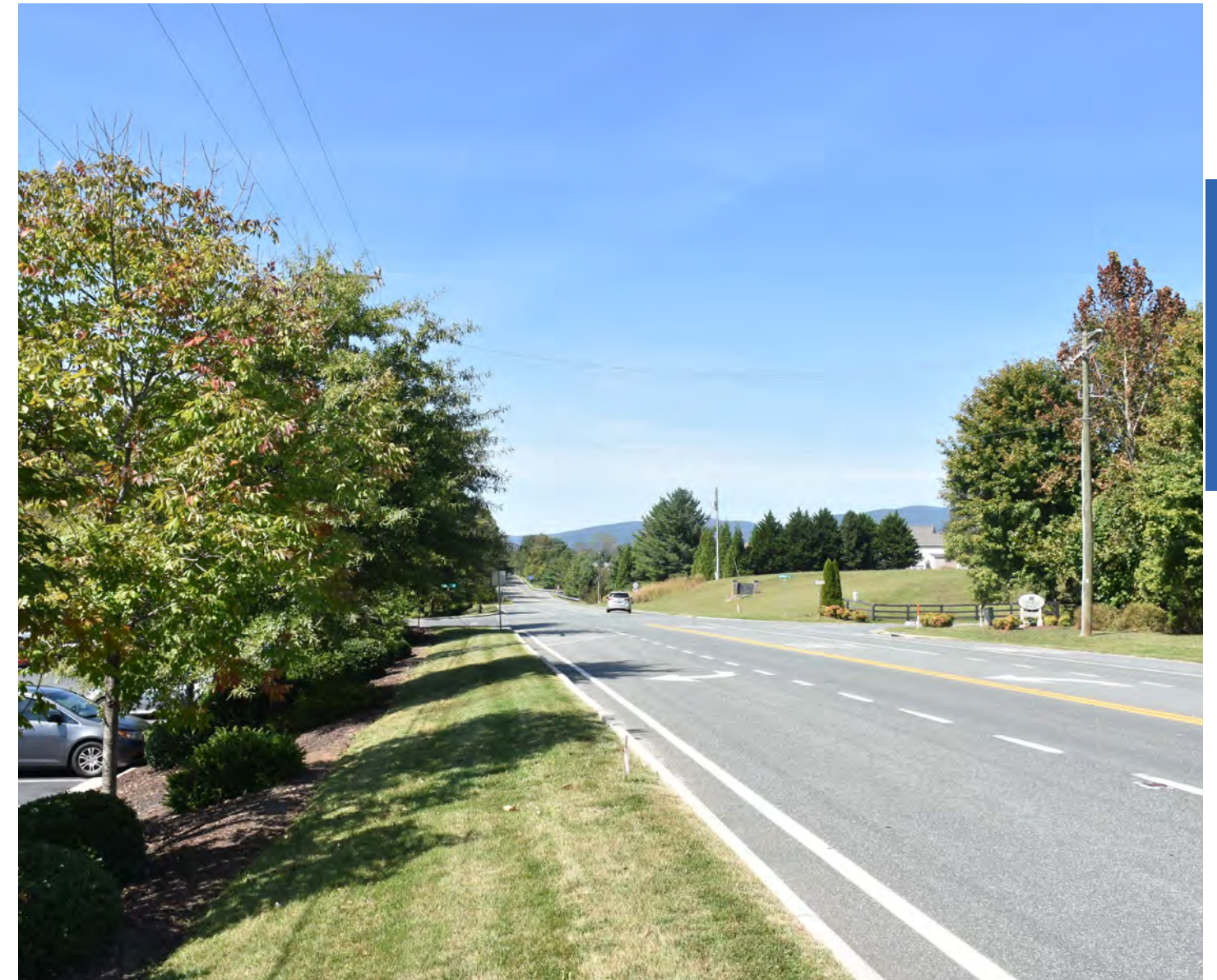
(Above) Route 250, alongside the Liberty Hall Neighborhood and Clover Lawn Village Center is the only Arterial in Crozet.
