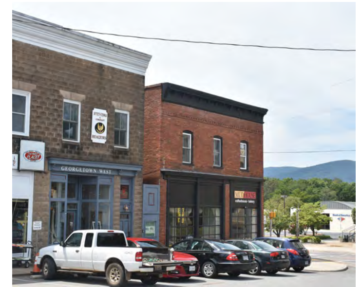
(Above) Existing buildings in Downtown Crozet that meet the form recommendations for live/work units.
