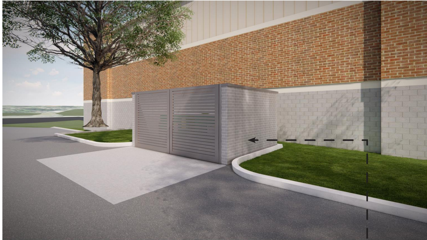
8' TALL CMU DUMPSTER ENCLOSURE CLAD IN GLEN-GERY THIN BRICK "FELDHAUS 800 CLASSIC GRAY SMOOTH" WITH WORKRITE MORTAR IN "WR-2055 GRAVEL"
