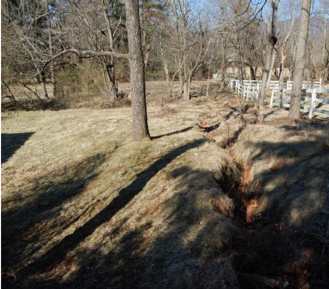
Pre-Restoration Photographs (Crozet Stream Restoration)
