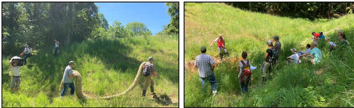
Stream Restoration Monitoring and Maintenance Training, May 27, 2021
