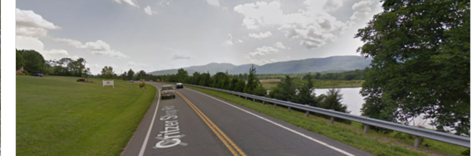
Vicinity of 9357 Critzer's Shop Rd.
