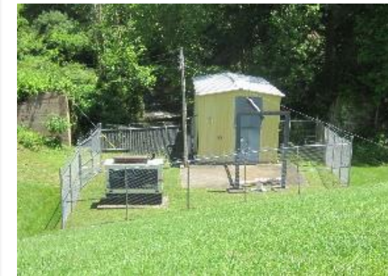
Existing Raw Water Pump Station to be demolished
