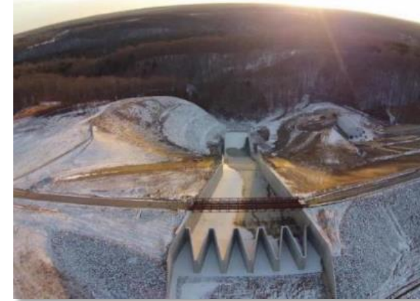
Proposed Labyrinth Spillway thru Dam with Bridge
