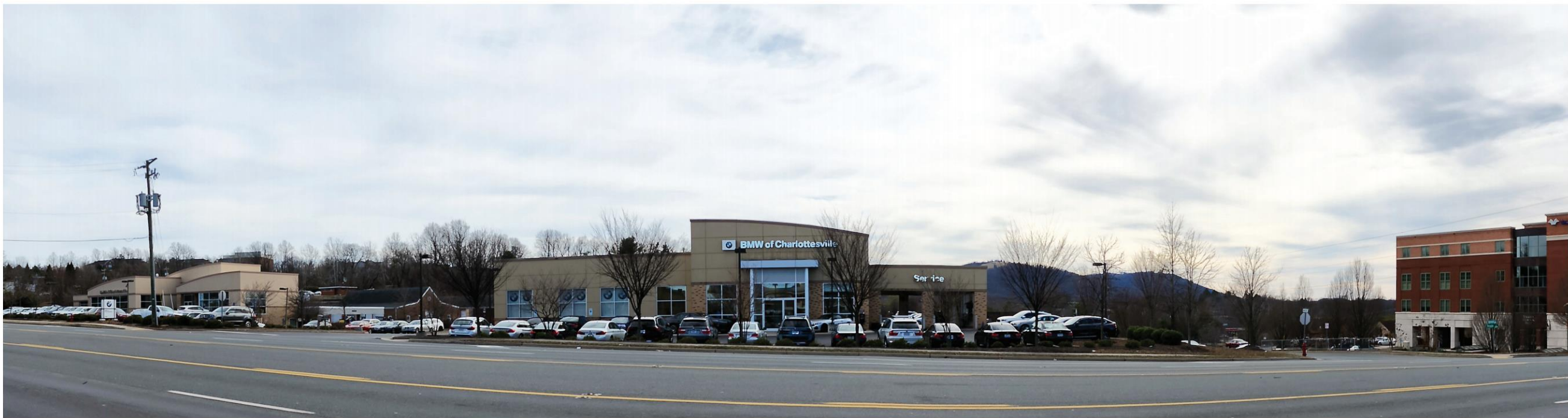
BMW EXISTING SERVICE BUILDING
