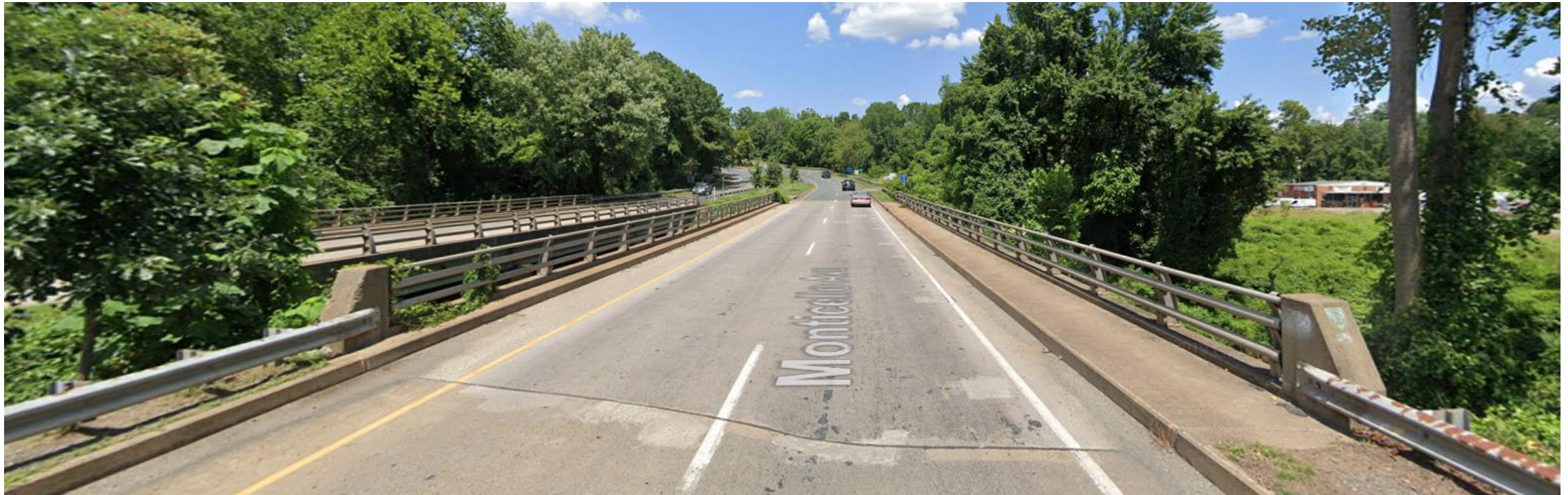
Width limitations imposed by bridge over Moore's Creek
