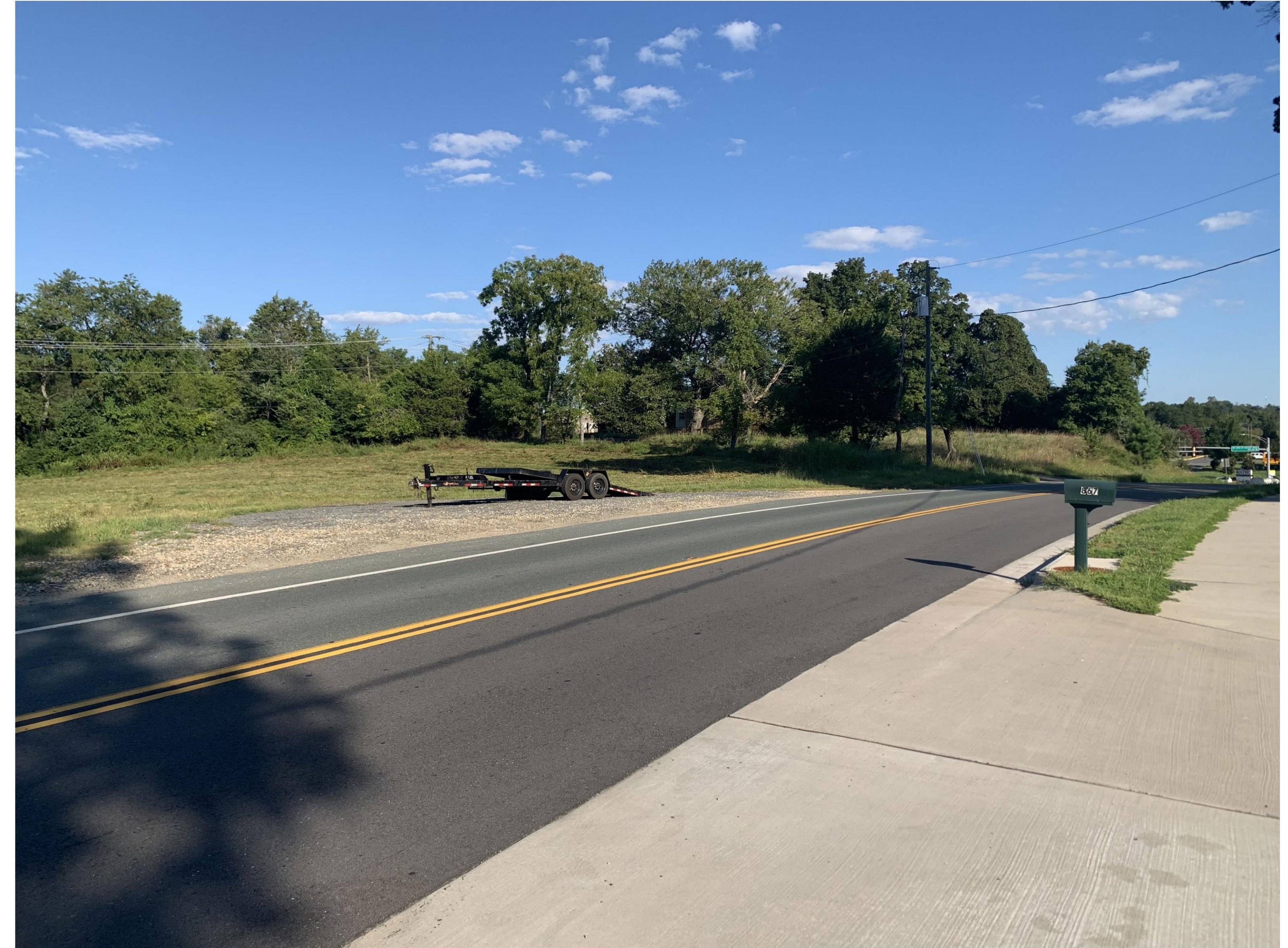
VIEW DOWN RIO ROAD EAST TOWARD INTERSECTION
