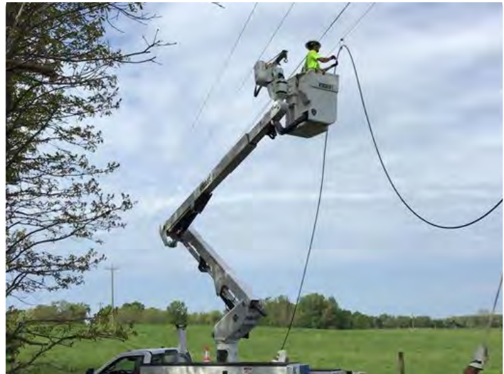
Fiber for broadband being installed along existing electrical infrastructure
