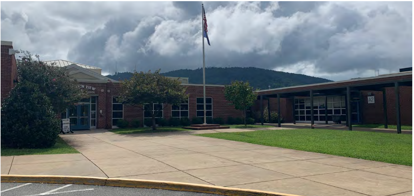
Mountain View Elementary School
