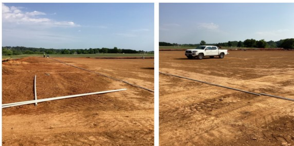
New Irrigation Being Installed at the Darden Towe Grass Fields.
