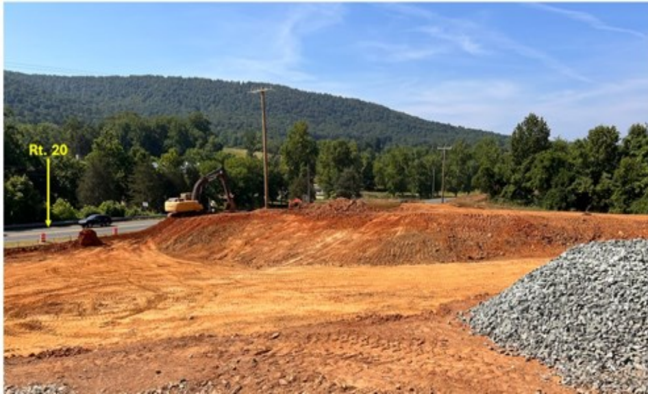
Biscuit Run Park Phase 1a Entrance Excavation
