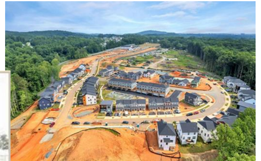
Southwood Phase 1: 211 units
