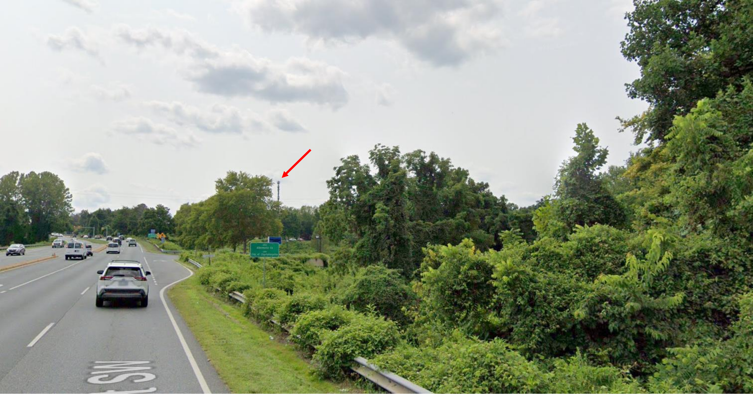
Existing Tower: View from 5 th Street Looking South
