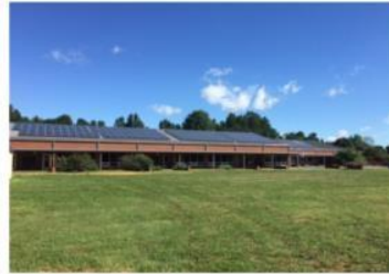
Rooftop solar installation at Brownsville Elementary School in Albemarle County.
