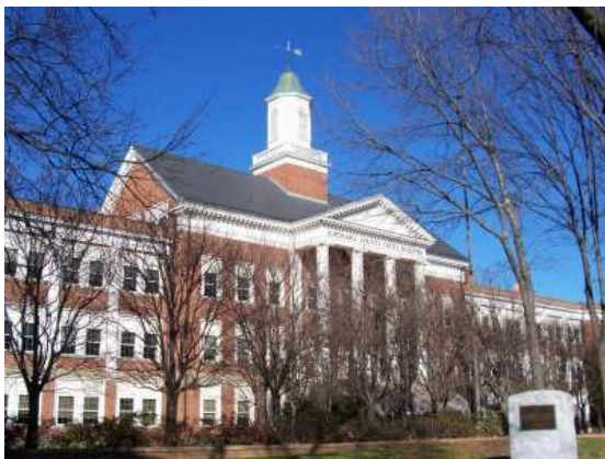
County Office Building, McIntire Road
