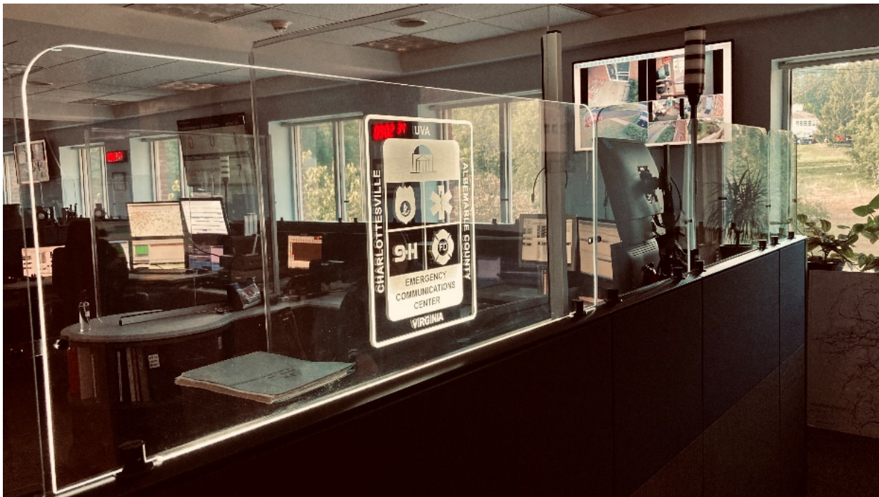
SCENES FROM ECC CONSOLE AND FLOOR REPLACEMENT PROJECT
