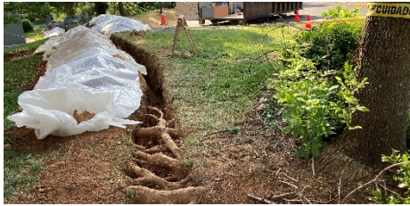
CONDUIT TRENCH WORK, IVY ROAD
