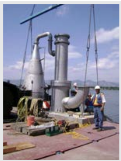
Speece cone to be submerged, Marston Reservoir, CO
