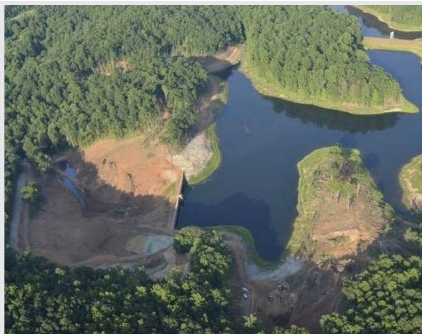
Aerial view of Ragged Mountain Reservoir during construction
