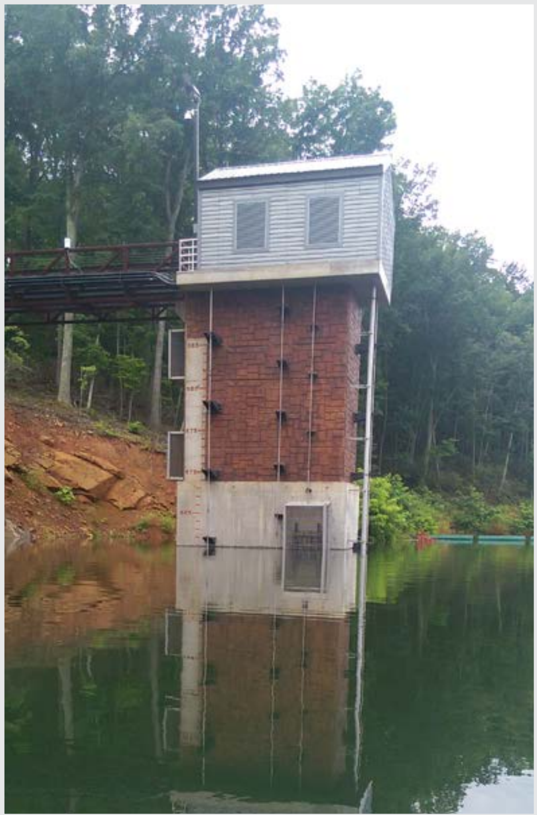
Ragged Mountain Reservoir intake tower July 14, 2015
