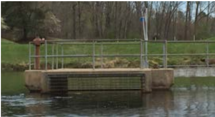
FIGURE 43. Beaver Creek Reservoir Outlet Tower at Full Reservoir Level
