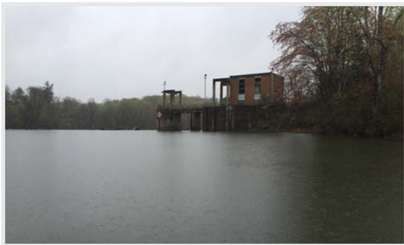
South Fork Rivanna Reservoir Outlet Tower, April 14th, 2015.
