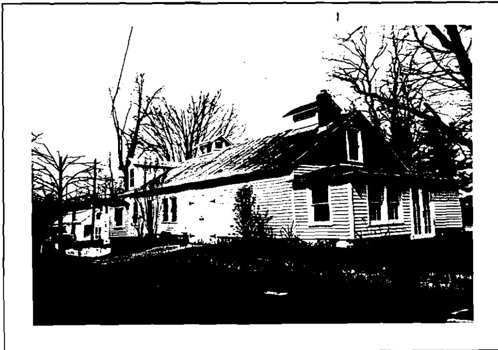
Figure 43. Ladd Blacksmith Shop (2-1061).
