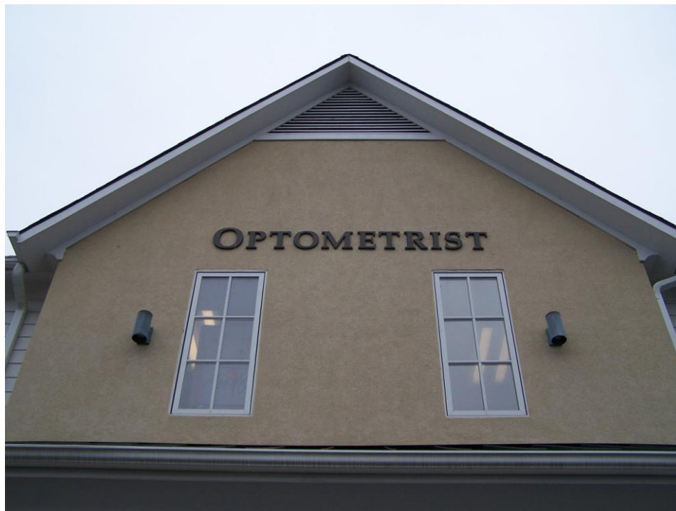
Sign #4: A bronze individually cut letter sign centered in a second floor gable.
