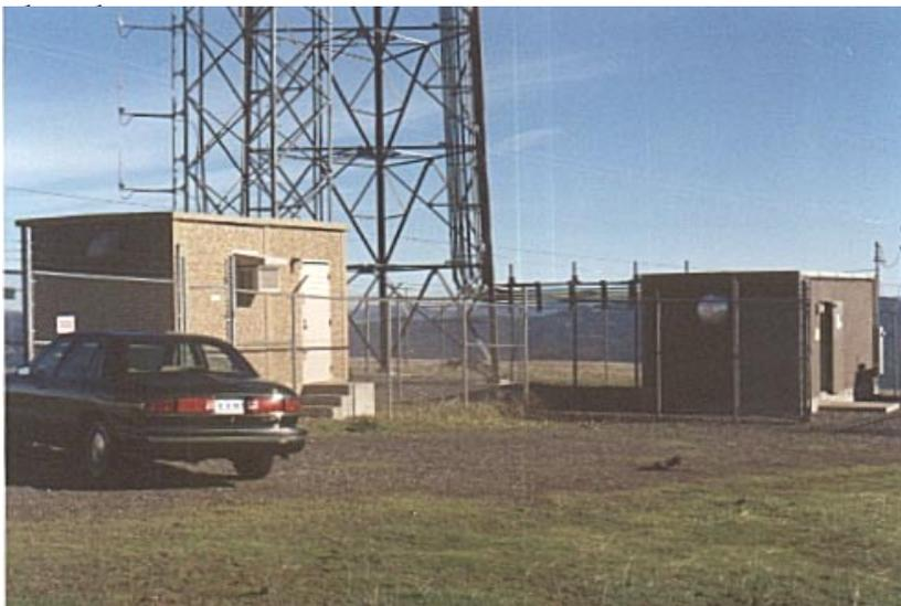
Equipment is often placed in small, pre-fabricated shelters or buildings. These two shelters for cellular facilities in Sonoma County, California must be air-conditioned. These types of facilities may not be acceptable in some locations due to visibility or other impacts on the adjacent areas.
