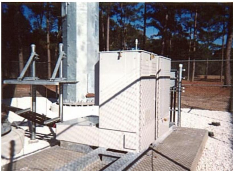
These two PCS equipment cabinets in Gainesville, Florida are smaller and lighter than cellular shelters. They do not need air conditioning. While less visible than facilities for cellular facilities, their visibility may be inappropriate in or near Avoidance Areas.
