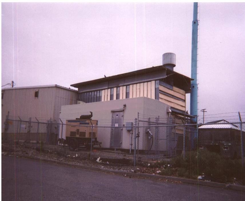
When the equipment area is large, or exposed, it should be buried in an underground vault. This photograph is an example of a cellular equipment shelter near a freeway in California. Only the maintenance cabinet is above grade.
