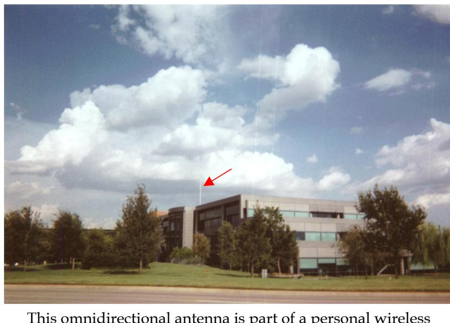
This omnidirectional antenna is part of a personal wireless service facility that is camouflaged as part of the GTE Headquarters in Irving, Texas. It could also be considered disguised as a flagpole, but it does not function as a flagpole.
