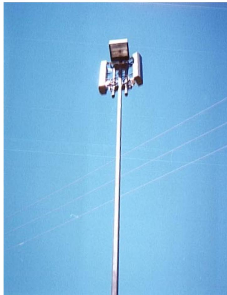
This personal wireless service facility has two dual-polarized antennas with a single floodlight.
