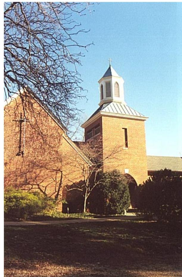
Personal wireless service facilities can be concealed in existing structures. The cupola of this church houses a personal wireless service facility. The original wood slats were removed and replaced with signal-transparent material.
