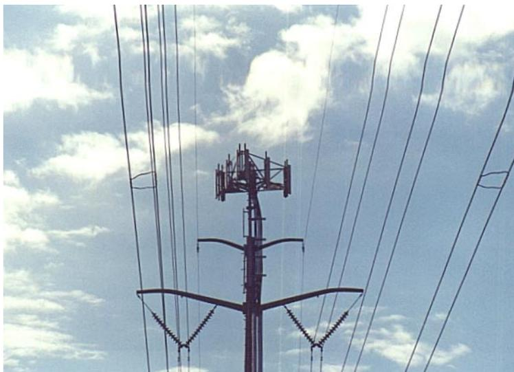
This antenna array on Barracks Road is sometimes called a “reindeer hat” or “top hat” array. These types of antennas can be found on transmission towers, lattice towers and monopoles.
