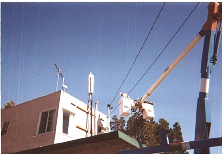
Dual-polarized personal wireless service facility being installed on the second floor of a motel in Marin County, California
