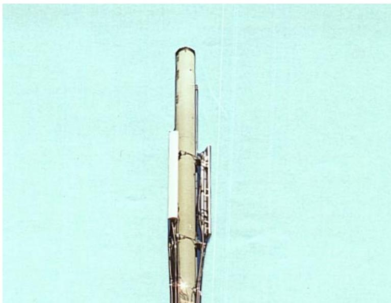
This is a dual-polarized or cross-polarized antenna on 5<sup>th</sup> Street. It can provide for polarization diversity and can do everything that the “top hat” array can do. Dual polarization eliminates the need for “spatial diversity”.
