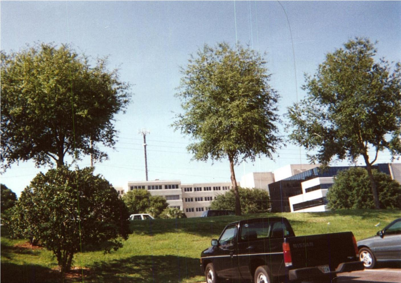
This personal wireless service facility in Florida looks like a monopole, but it isn't. Guy wires hold up the lattice mount. It is a guyed tower on the roof of a hospital.
